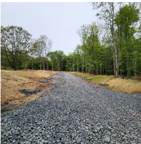
Stabilized Construction Entrance and Check Dams
