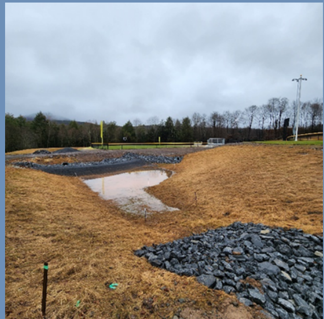
Sediment Forebay and Infiltration Basin at Catskill Mountain Little League Field
