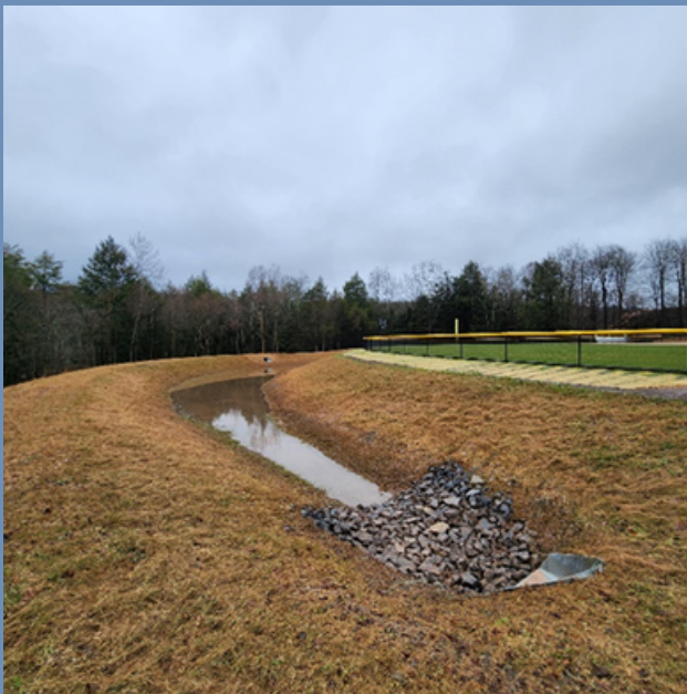
Sediment Forebay and Infiltration Basin at Catskill Mountain Little League Field
