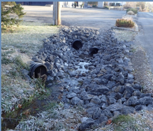
Rip Rap Drainage Outlets
