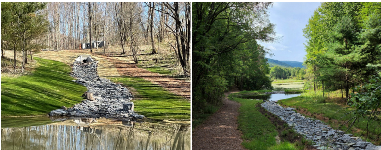
Outlet Drainage Structure to Sediment Fore-bay
