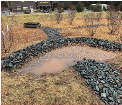
Forebay and bioretention basin in Neversink
