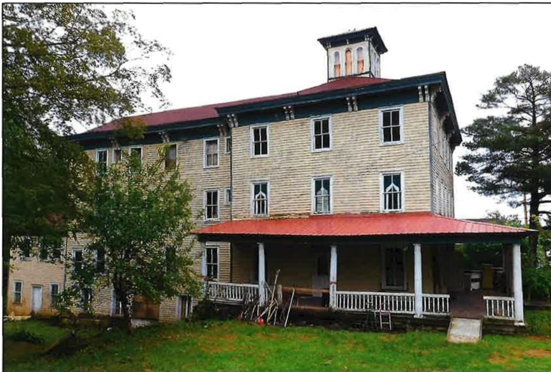
Fig 00.04: West elevation, front block, looking east
