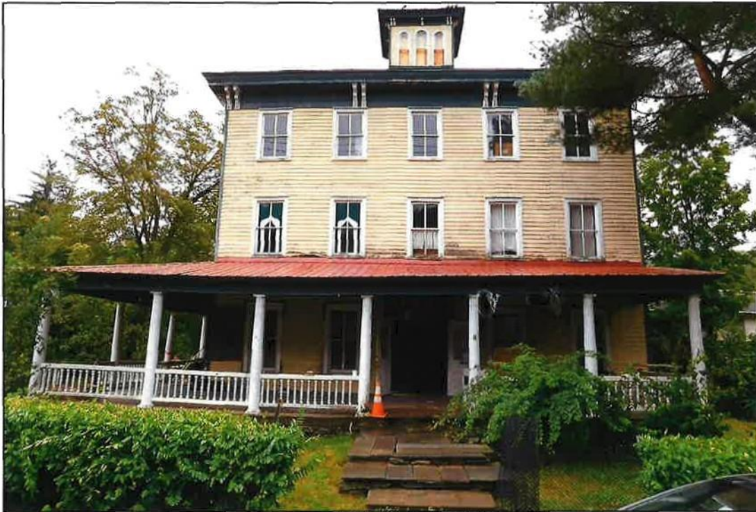
Fig 00.03: South elevation, looking north
