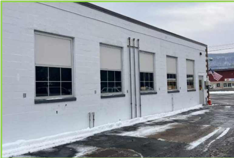
West side of the building
