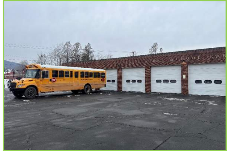
Front side of the building
