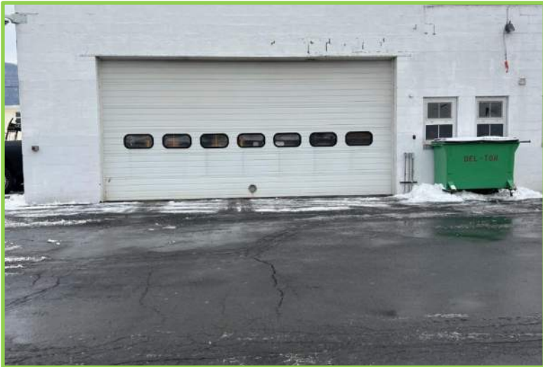
North side 22-foot garage door
