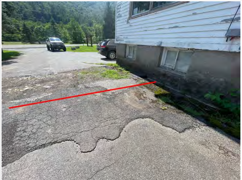
White House: Location of existing sewer line noted
