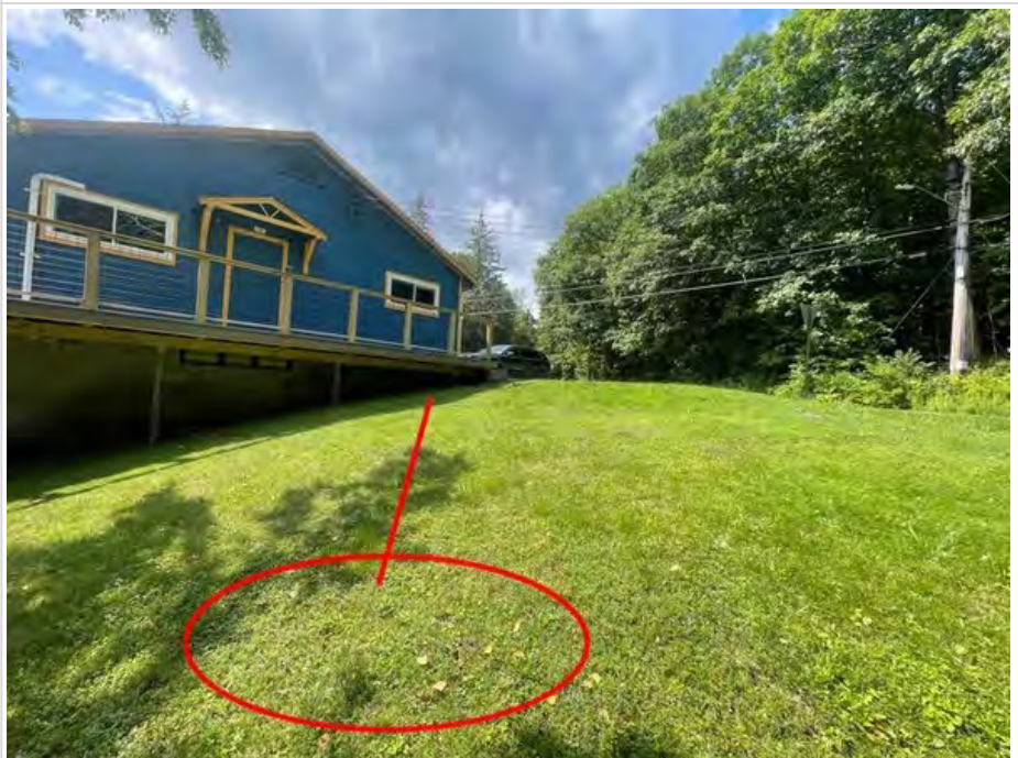
Red House: Sewer line and location of 1500gal tank noted
