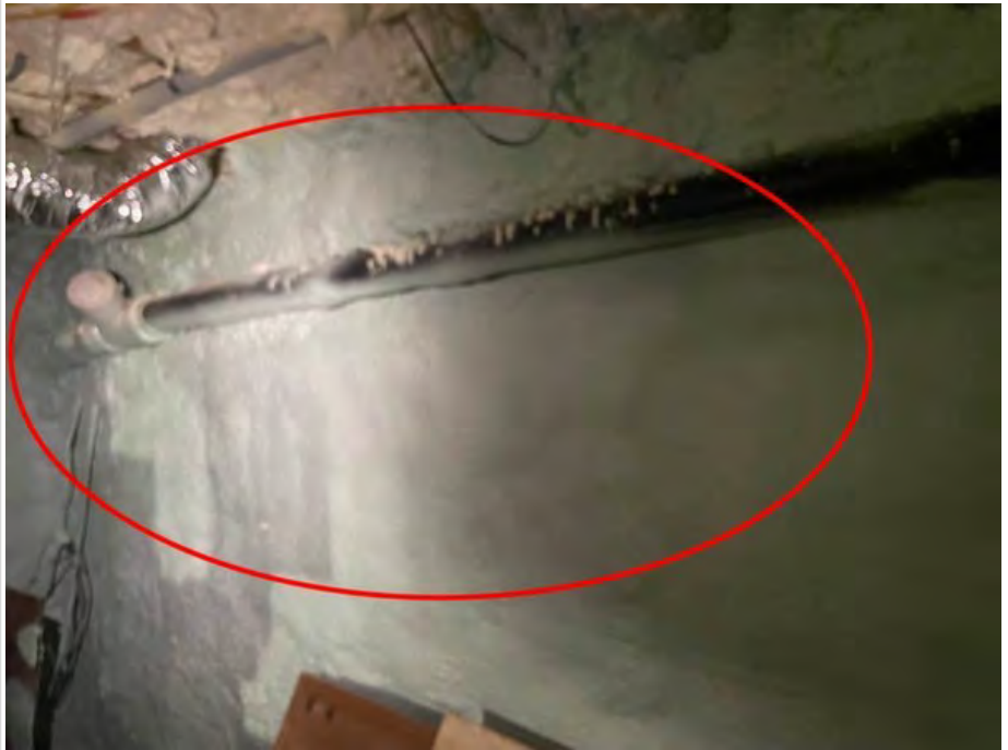
Red House: Existing sewer line
