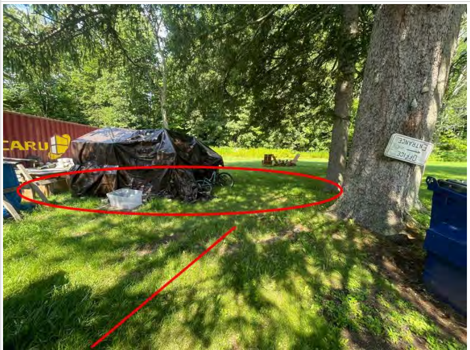
White House: Location of pump tank 2 & 2500 gal septic tank
