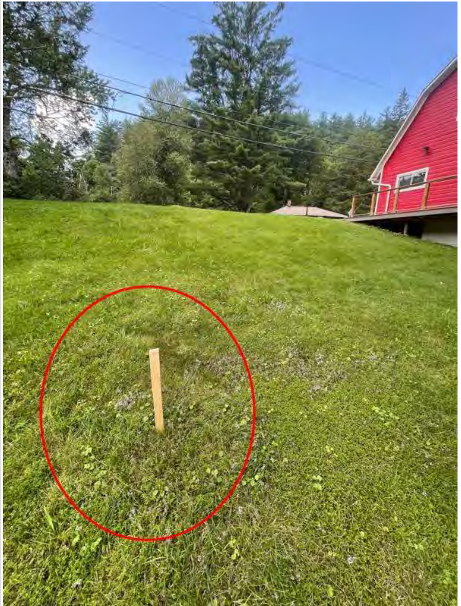
Blue House: Site facing W. Location of pump tank 1 noted
