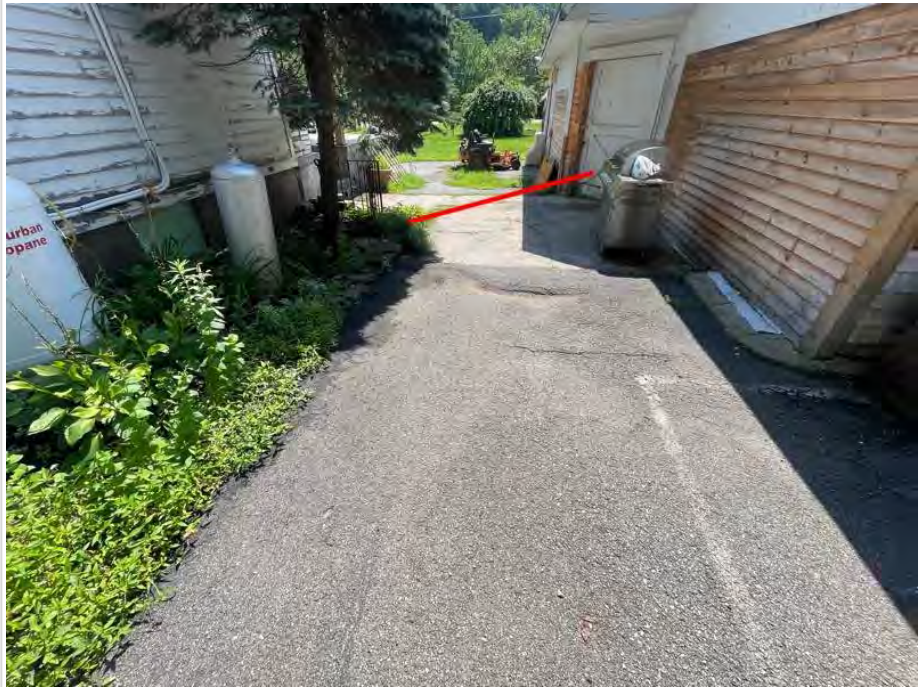
Caretaker House: Sewer line noted
