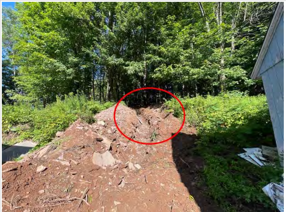
Site facing NW. Pump line installation progress notes
